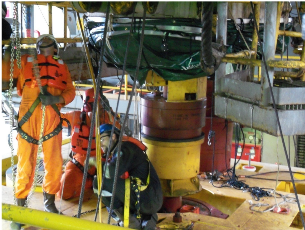
Pulling caisson BC-10.
