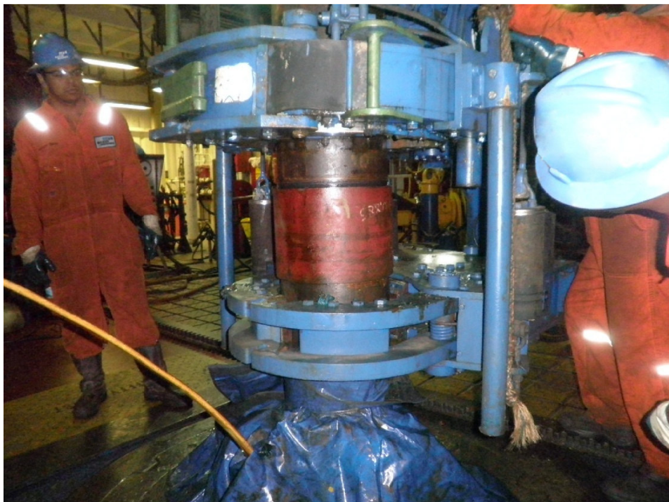
Tong and backup breaking connection.
