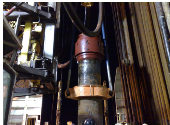
Figure 9: 32-in. caisson being run with 32-in. elevators.
